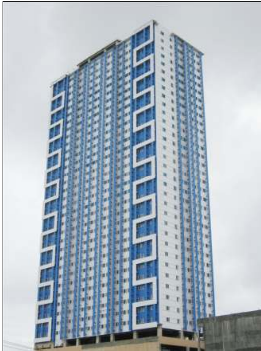
View from Gilmore Avenue (Rear)
